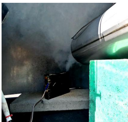
Figure 97. The battery venting into the fire hood.
