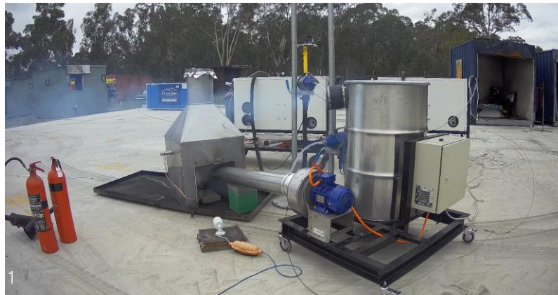
Figure 96. The scrubber testing configuration.
